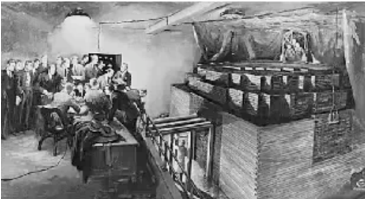
Control of the reactor with cadmium bars.
